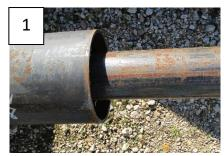
1. **Preparation:** Remove dirt and debris from Casing end and Carrier where End Seal will be installed. Measure and note the actual Casing size and Carrier size.
