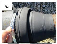
5. **Tighten Clamps:** For both ends, flip up clamp screw and feed threaded portion of band under screw. Pull band snug (5a) and flip down clamp screw. Tighten clamp (5b) screw using a 5/16" socket or flathead screwdriver until end seal is securely fastened to Casing and Carrier.
