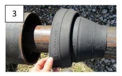
3. **Position on Casing and Carrier:** Slide over Carrier and onto end of Casing. Assemble worm gear bands on Casing and Carrier over End Seal ends for tightening.
