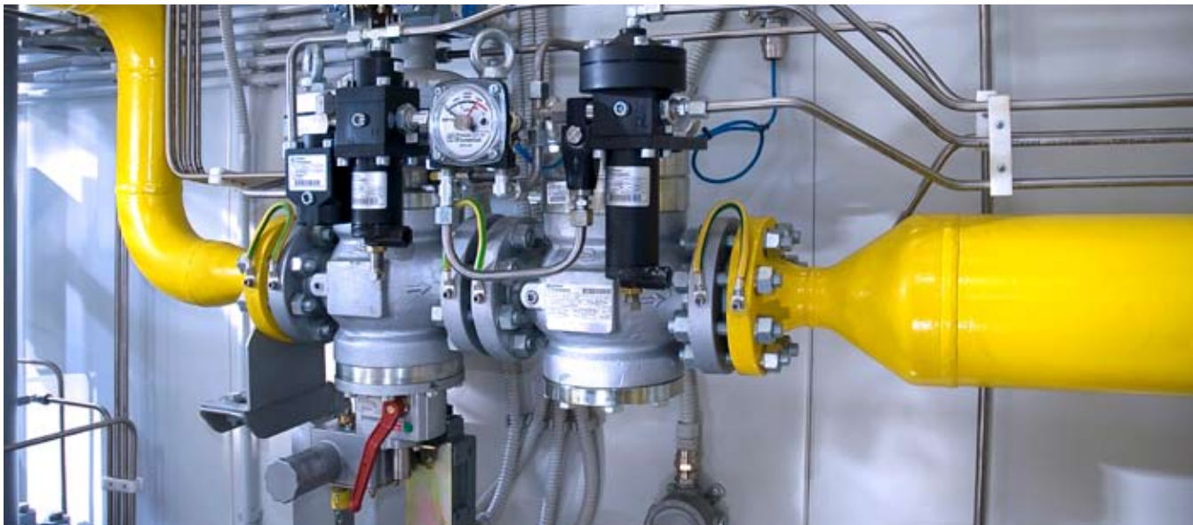
Aperflux 851 pressure regulators in action
