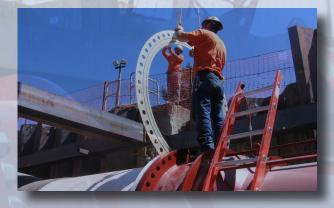
Trojan gaskets are state-of-the-art, with near zero leakage static sealing. The elastomer sealing element is encapsulated in the electrically isolating retainer. The
