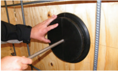
1. Extend (threaded rod*) through form and first locator cap and (threaded nut*) on the back side of form.
