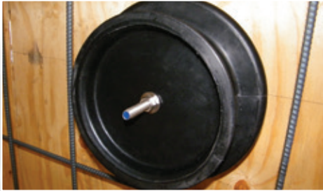
3. Slide second locator cap through (threaded rod*), use fender washer and fasten nut until locator caps and sleeve are locked in place. Check to make sure sleeve is square to form.
