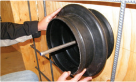
2. Attach Infinity® wall sleeve to locator cap.
