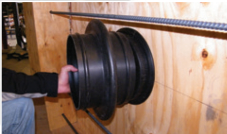
3. Cut the Infinity® wall sleeve 3/4" shorter than the wall thickness (+/-1/4"), then insert the sleeve over the locator cap.
