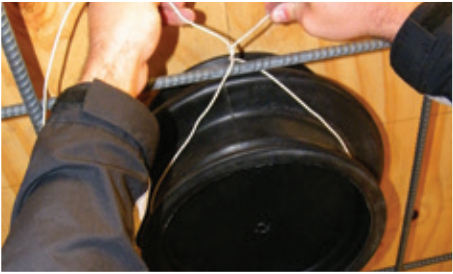
5. Attach the Infinity® wall sleeve to the rebar using wire.
